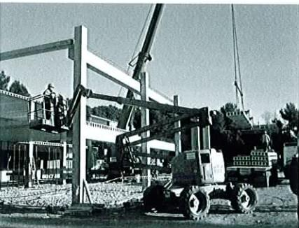
*The structural frame consists of pieces that were brought in directly from the factory. The size of the bay makes it possible to optimize the length of the beams that, supported by pillars built into the floor through on-site footings, also serve to hold up the slab of alveolar plates that have 30-centimeter edges.*
